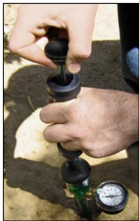
De-airing in the Ground
